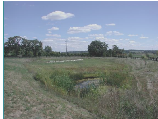
DNR Photo. Infiltration and bioretention basin.
