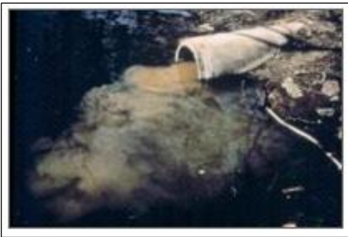
DNR: Storm sewer outfall discharging sediment to a stream.
