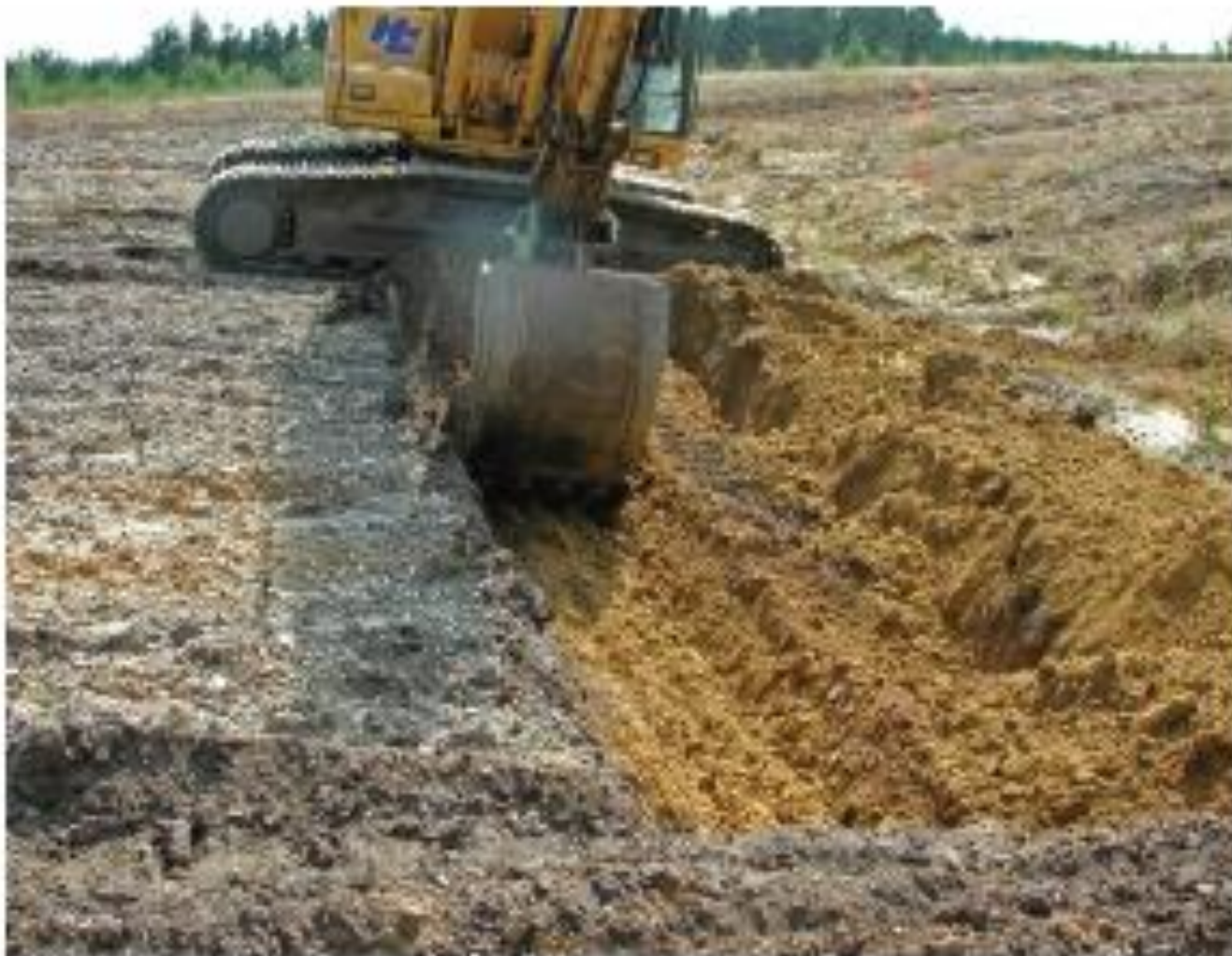
Figure 1 An excavator removing soil.
