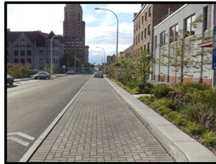
Porous paver parking lane with bioretention garden.
