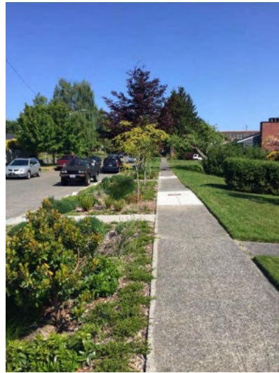
Residential rain gardens with porous sidewalk.
