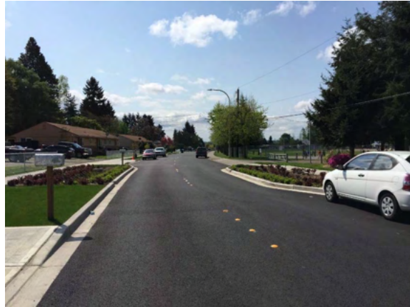
Residential setting bioretention with curb bump outs.
