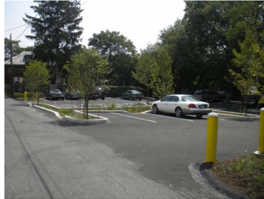
Parking lot with bioretention.
