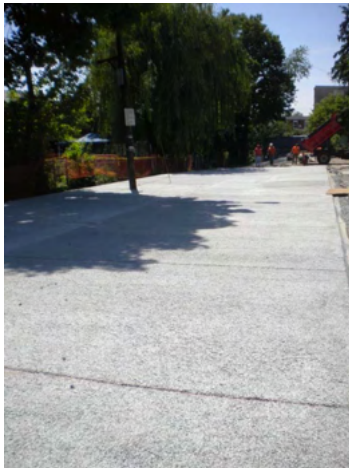
Parking lot with porous pavement and bioretention.
