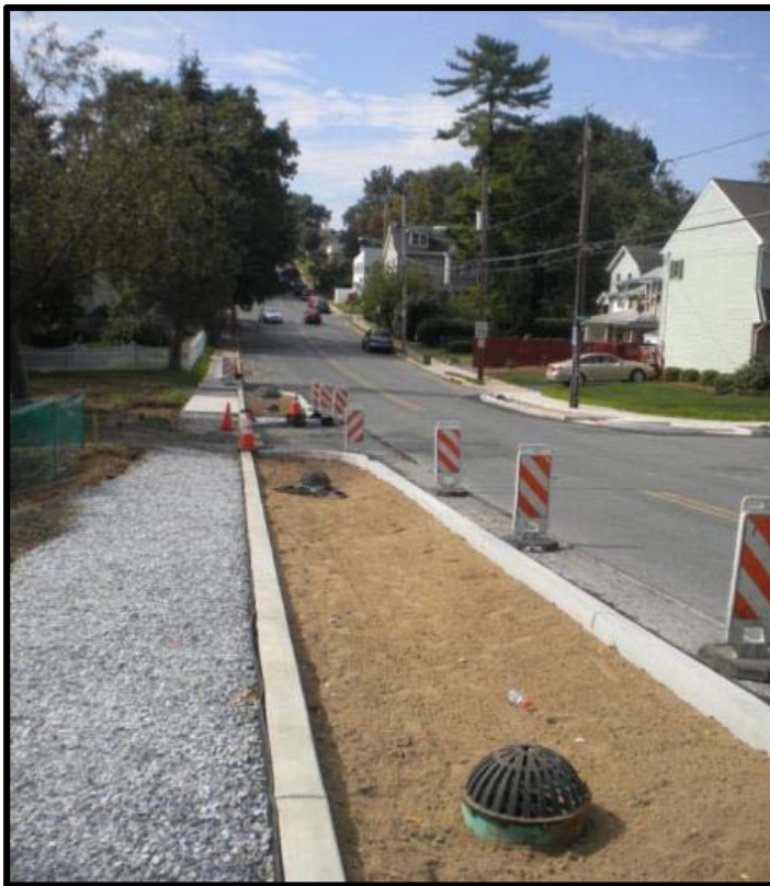
Curb bump outs in residential neighborhood create bioretention garden.
